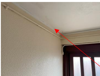
Plastic trunking on ceiling.
