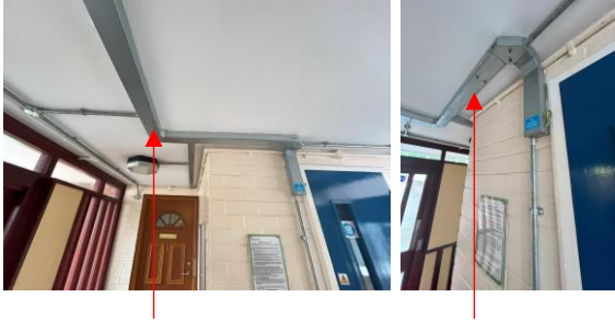
Metal Electrical Trunking
