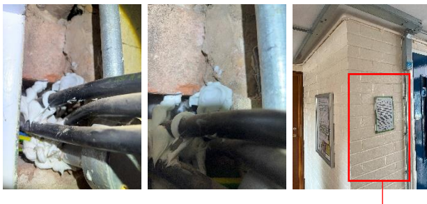
Fire stopping required Area of where cables run through.
