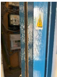
FD30s fire rated doors are used for the electrical cupboards.
