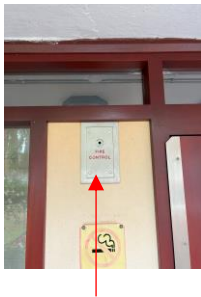
Firefighters Override Switch
