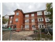
2)uPVC double glazed units have been installed to each flat and communal stairway. There is a porched entrance to the block. The canopy roof is a pitched roof with flat interlocking roof tiles. There is uPVC facia and soffits installed around the porch front. Entrance & rear door are timber and glass units, with small section of spandrel panelling to the side. The bin room door is of timber construction.
