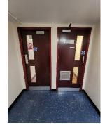
8) The door to the bin store from the ground floor lobby is FD30s and is additionally fitted with a ventilation panel with intumescent baffle.
