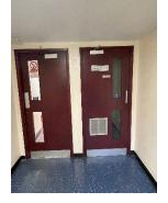
Each block has its own bin store adjacent the main entrance with access for residents via an access hatch which is further separated from the ground floor lobby via an FD30s fire door with vision panel and intumescent baffle.
