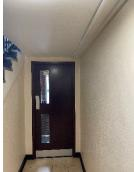
9) The final exit doors to the front of the building have door entry systems installed. These systems are designed to fail safe i.e. door unlocked in the event of a power failure. This prevents residents being locked in or out of the building. All final exit doors are openable by means of a levered handle.
