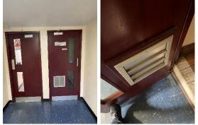
9) The cleaner's cupboard in each block has a timber FD30 door secured with a suited type 54 mortice lock and is located on the ground floor between the rear final exit door and communal door to the lobby.
