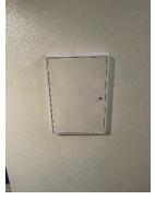
16)Fire resisting hatch (block 13-18) does not fully close into frame.
