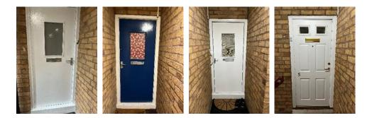
12) Accessed Flat 3 has no self-closing device and no intumescent strips or smoke seals. The door is a appears to be a replacement notional fire door (FD30 label present) There is a 10mm door stop. A selfclosing device and intumescent strips and smoke seals are required to be fitted. Resolved.
