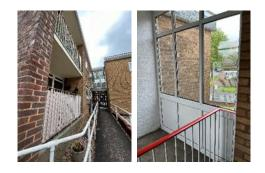
Individual flat windows are UPVC double glazed window frames. Windows in the common area stairwell have spandrel panels. The windows in the communal staircase area are UPVC window frames with small trickle vents only.
