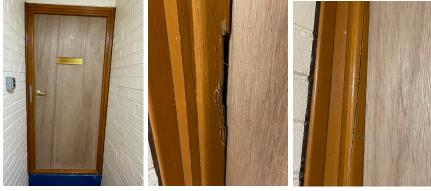
B. Flat 8 has a temporary timber flush fire rated door. (access not gained for internal inspection)
