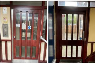
6) The final exit doors have door entry systems installed. These systems are designed to fail safe i.e. door unlocked in the event of a power failure. This prevents residents being locked in or out of the building.
